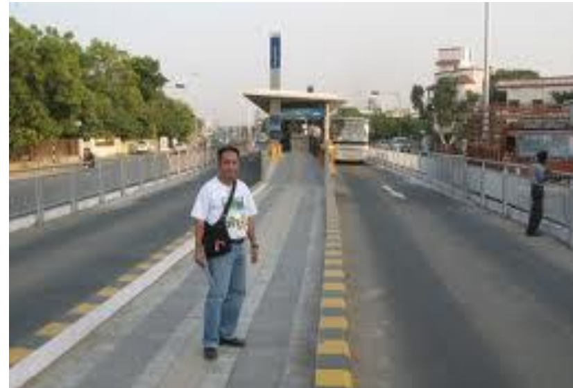
Picture 5-7: Continuous footpath to access to BRT shelter, BRTS, Ahmedabad
