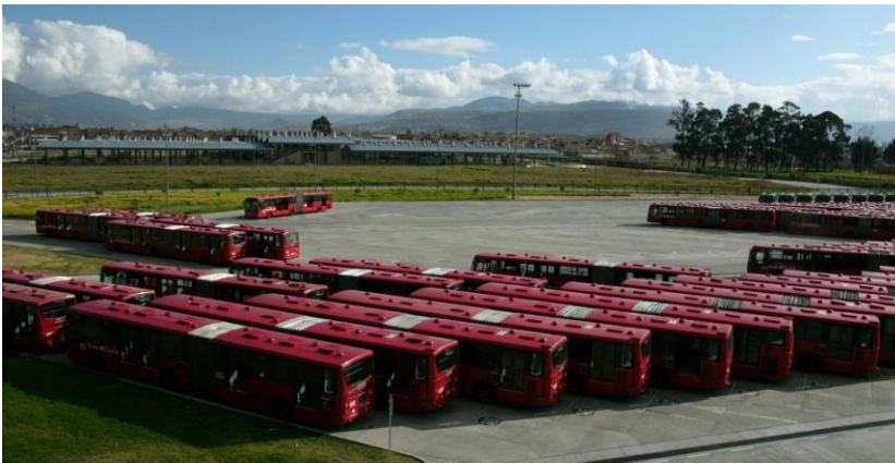
Picture 7-3: Terminal cum depot facilities, BRTS, Curitiba, Brazil
