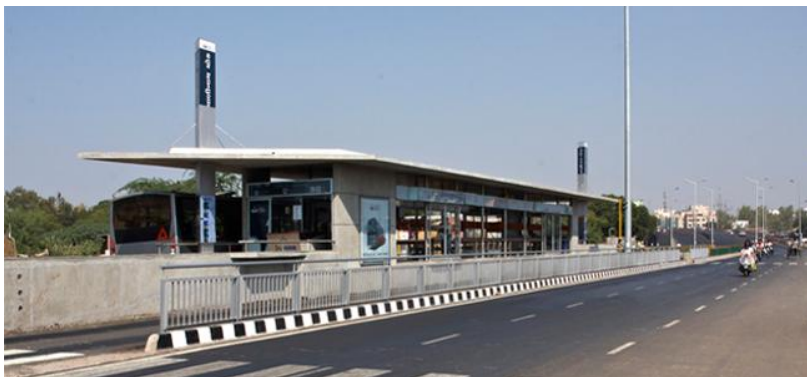
Picture 4-2; Enhanced Bus Stop, BRTS, Ahmedabad
