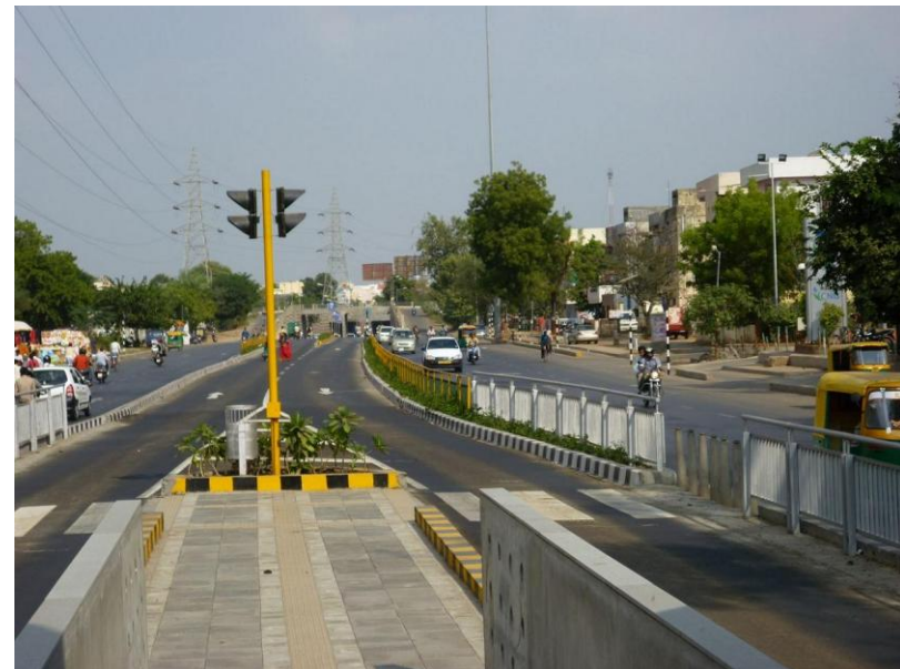
Picture 5-5: Refuge island and at-grade access to BRT shelter, BRTS, Ahmedabad, India
