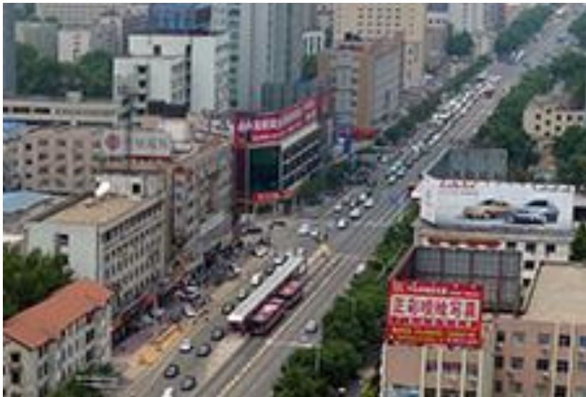
Picture 4-29: Far side BRT bus Station, BRTS Zhengzhou, China
