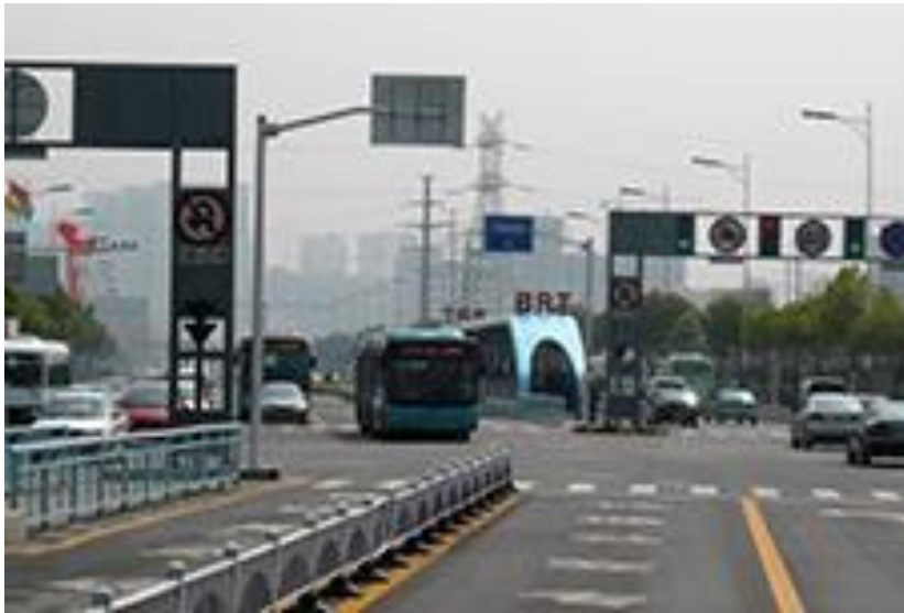
Picture 4-30: Near side BRT bus Station, BRTS Changzhou, China
