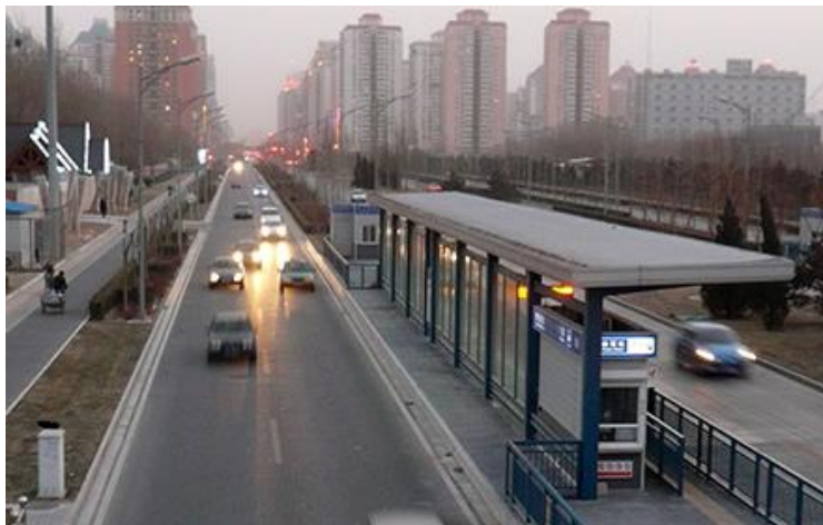
Picture 3-17: Flexible Pavement in Beijing BRTS, China
