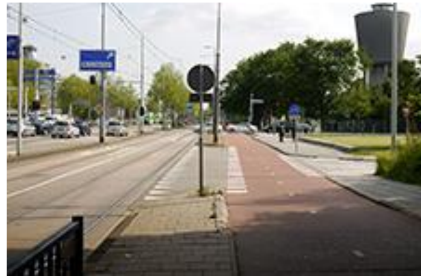
Picture 5-8: Refuge Island facilities for access to BRT shelter, BRTS, Kunming
