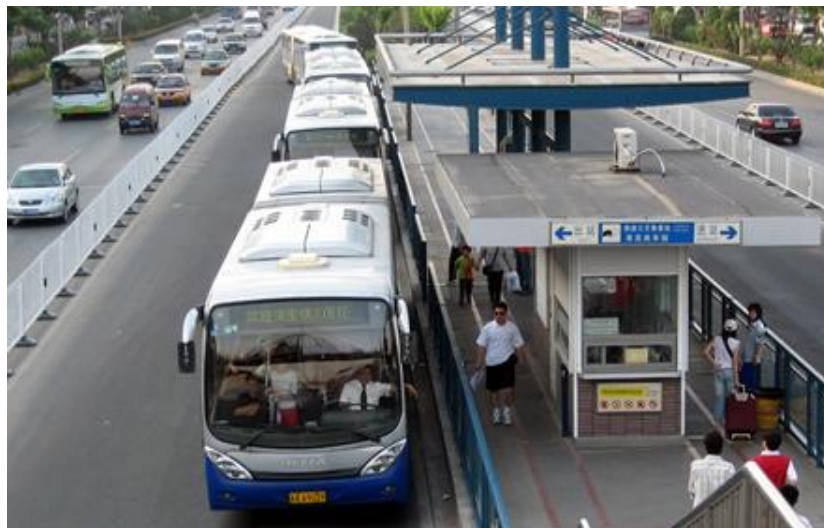
Picture 5-2: Continuous footpath and grade separated access to BRT shelter, BRTS, Beijing, China
