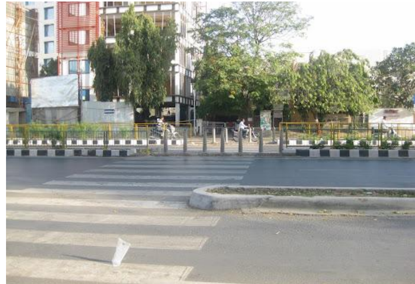
Picture 5-6: Pedestrian crossing for access to BRT shelter, BRTS, Ahmedabad
