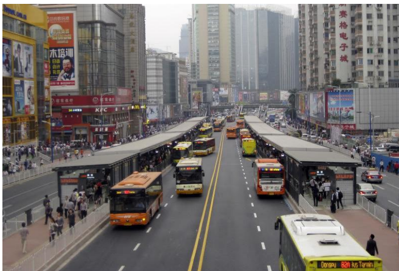
Picture 4-13: Extended Bus Platform with unassigned berths, china
