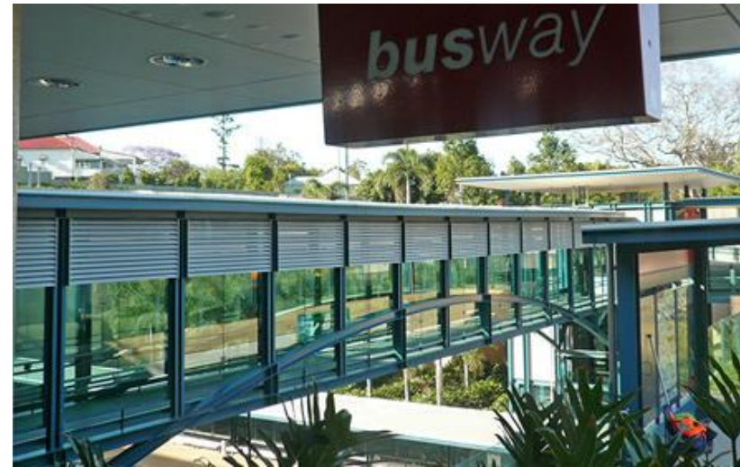
Picture 5-3: Grade separated access to BRT shelter, BRTS, Brisbane
