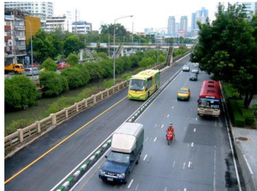
Picture 3-14: Flexible Pavement in Bangkok BRTS, Thailand
