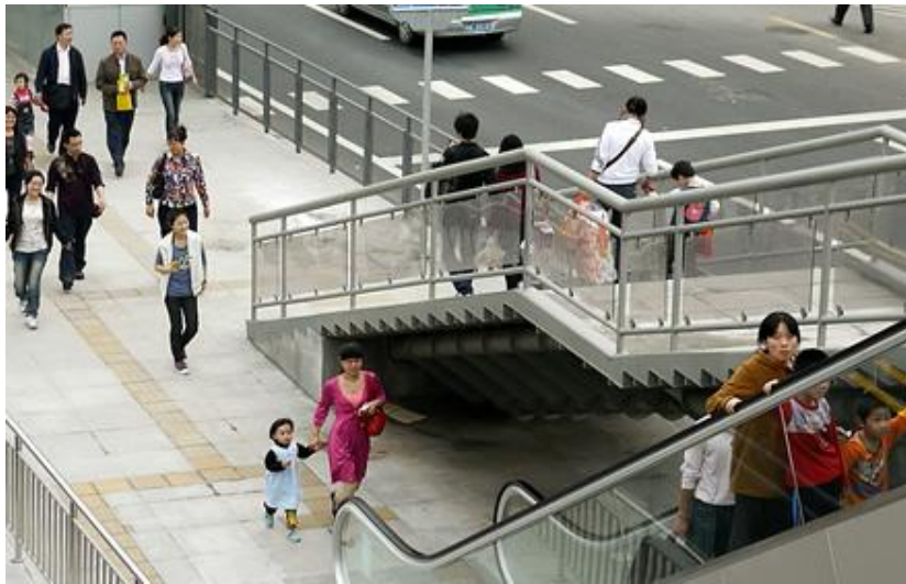
Picture 5-4: Continuous footpath and grade separated access to BRT shelter, BRTS, Guangzhou, China
