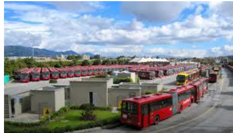
Picture 7-4: Terminal cum depot facilities, BRTS, Bogota, Colombia, SA
