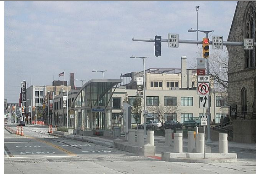
Picture 4-22: Curb side station
