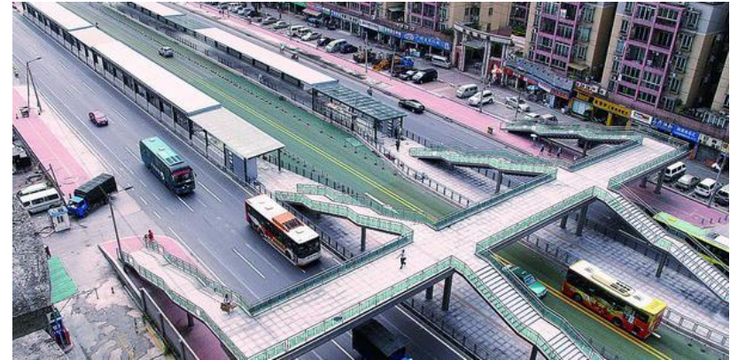
Picture 5-10: Grade separated pedestrian foot over bridge to access the BRT shelters, BRTS, Guangzhou, China
