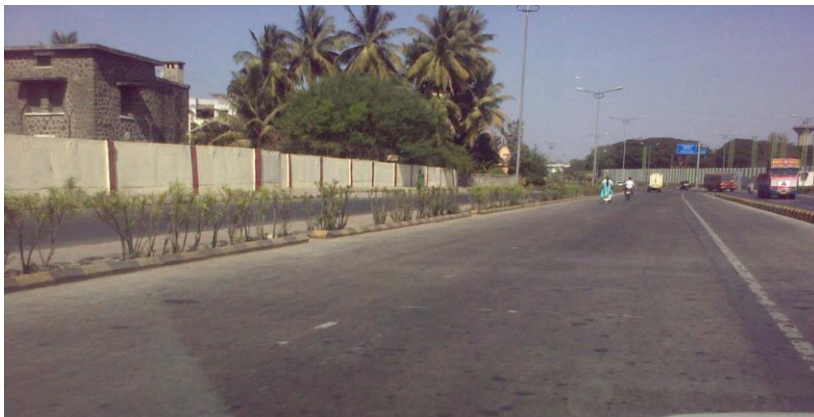
Picture 2-6: Alandi Road (Corridor 2)
