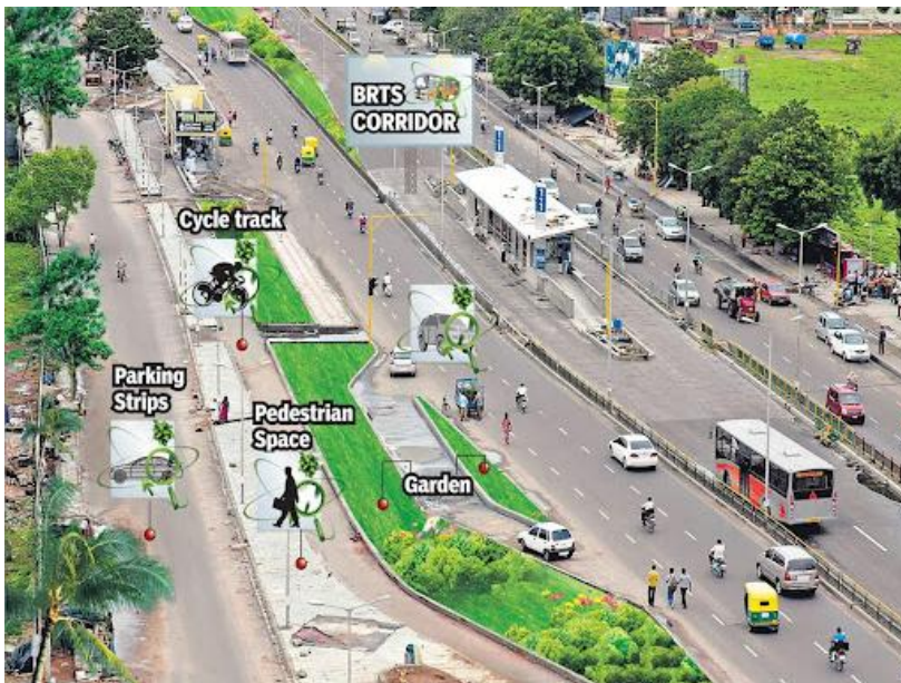
Picture 6-1: Provision of Parking facilities near BRT shelter, BRTS, Ahmedabad, India
