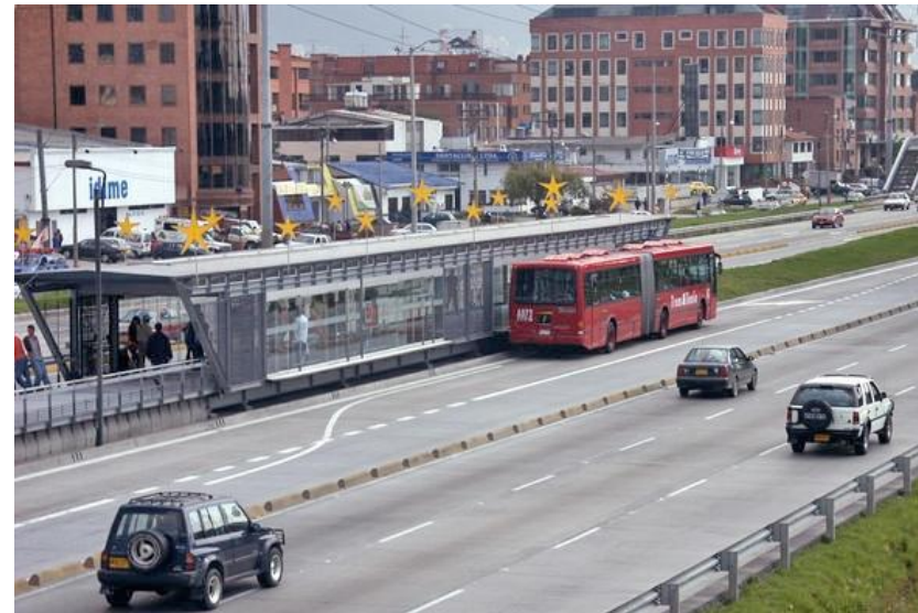
Picture 4-31: Mid Block BRT bus Station, Bogota, Colombia
