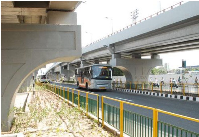
Picture 3-12: Lane delineators in Ahmedabad BRTS
