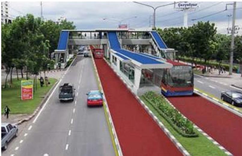
Picture 5-11: Pedestrian foot over bridge facilities for access to BRT shelter, BRTS, Bangkok, Thailand
