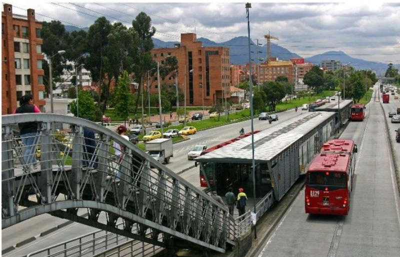
Picture 4-24: Median side station with median side platform, BRTS Bogota
