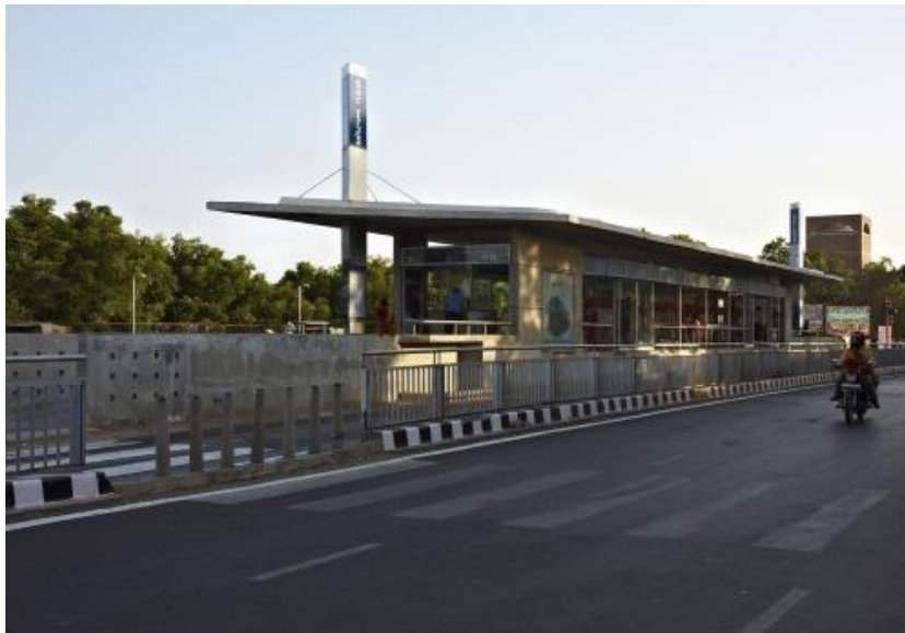
Picture 4-19: At Grade station access to BRT station, Ahmedabad BRTS
