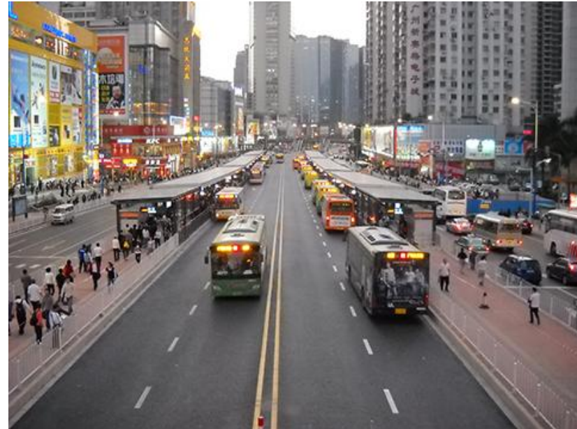
Picture 4-23: Curb Side Station on Median Bus Lane, Cleveland Health Line
