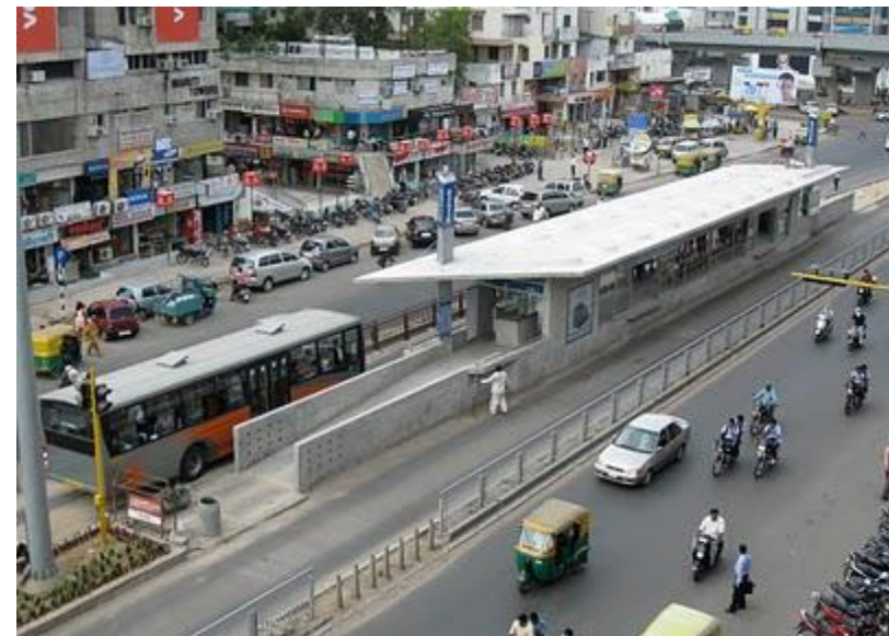
Picture 4-14: Station with no passing lane, Ahmadabad BRTS
