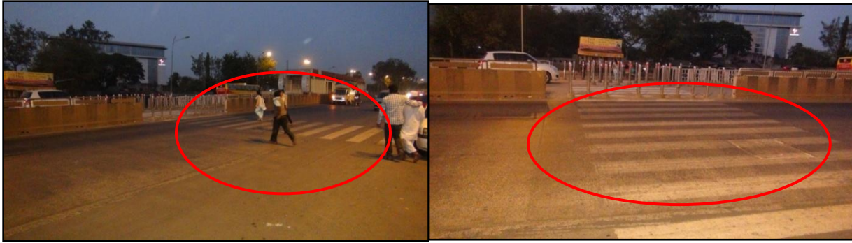
Observation 59: Absence of reflectors and separate signal for BRTS near IBIS hotel
