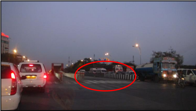
Observation 59: Absence of reflectors and separate signal for BRTS near IBIS hotel
